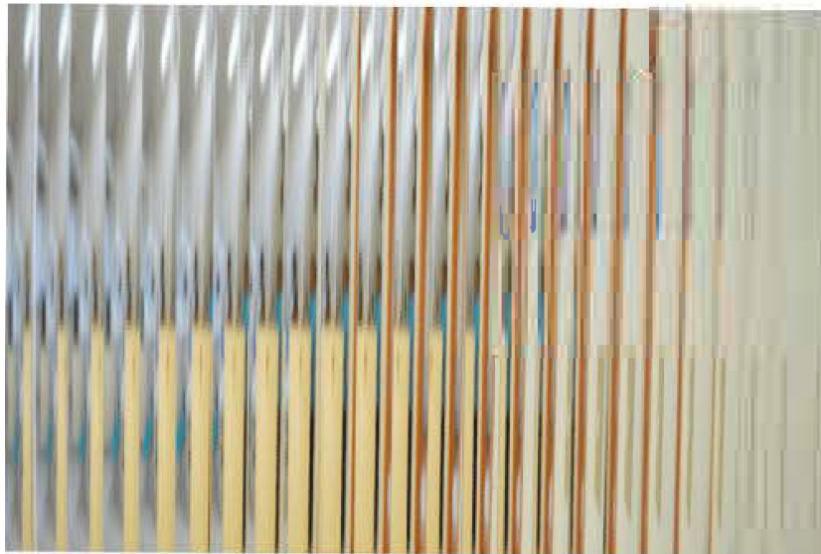
Glass partition with fluted glass for privacy covered with thin metal frame.
